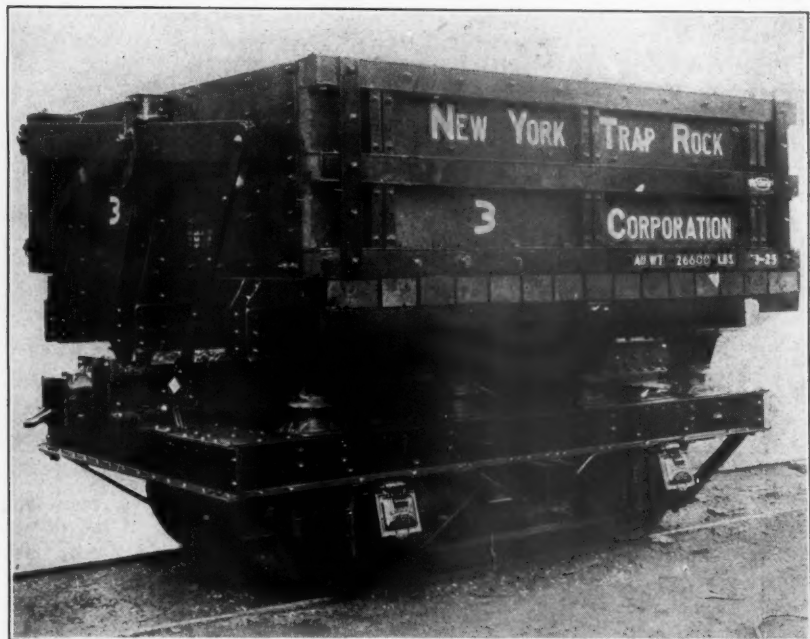
Western Dump Car Operated by Electricity
